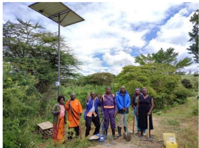
Completed solar pump well
