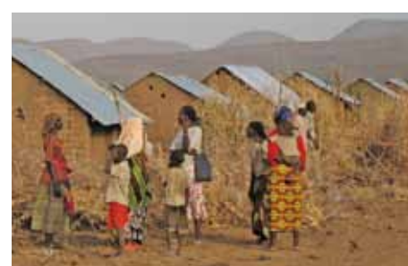
New homes in the desert: PWRDF funded 150 homes at Kakuma Refugee Camp.
